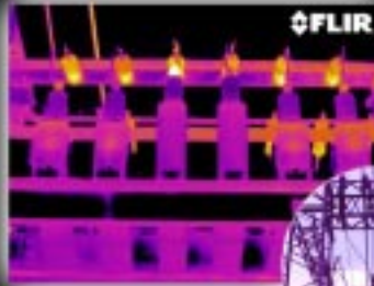
Bad connections on a capacitor bank
