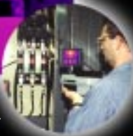
Connection problem on 200 Amp fused disconnect
