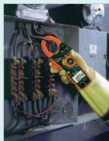
CAT IV -600V safety rating for added protection and True RMS feature gives you accurate readings of non-sinusoidal waveforms.
